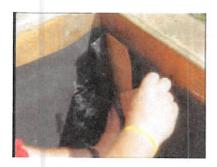
**Step 5**- Remove the release paper and adhere the PondGard flap to this Splice Tape to create a sealed seam.
