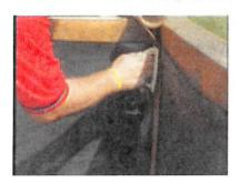
**Step 4**- Adhere the 3.00" (7.62 cm) QuickSeam™ Splice Tape to the primed surface of the bottom panel.
