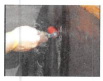
**Step 6**- Using a hand roller; roll the seam to ensure adhesion at all points.
