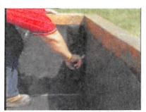
**Step 3**- Test the primer flash-off by touching the primed area with your finger and pushing forward at an angle. The primer should not string as your finger is moved up and away.
